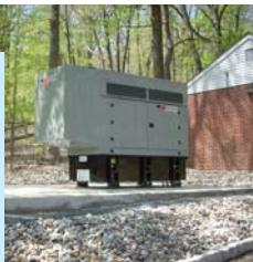
The Jockey Hollow Booster Pump Station, located on Western Avenue in the Township of Morris, was completely rehabilitated in 2012. An antiquated standby generator was replaced with a new, fuel efficient, air emissions compliant diesel powered unit. The pumps and control valves were replaced. Also, new energy efficient motors and controls were installed.
