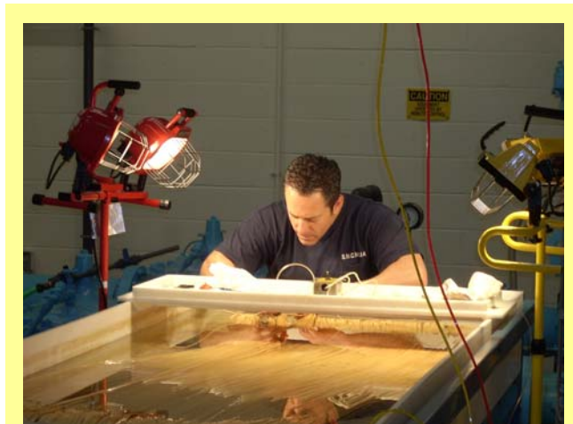
SMCMUA Treatment and Pumping Apprentice Operator Repairing Membrane Fibers Used to Filter Water at the Clyde Potts Reservoir in the Township of Mendham
