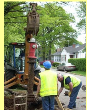
SMCMUA's Transmission and Distribution Personnel Installing a Fire Hydrant
